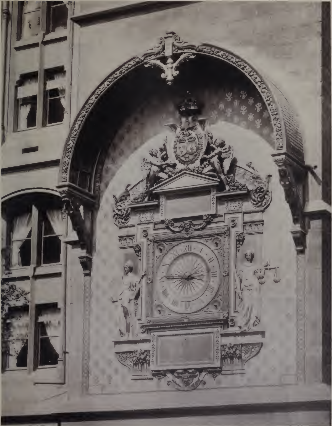
11A. ORNAMENTAL CLOCK TOWER FACADE
